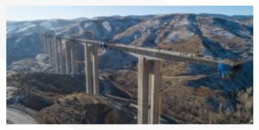
The tender related to the Eyiste Viaduct has been carried out by General Directorate of Highways. The contract has been awarded to Nurol Construction at end of 2016. Within the scope of the Project, a viaduct with a total length of 1,372 meters and a width of 25 meters will be constructed; and it will be one of the world's biggest balanced cantilever viaducts. The superstructure will be constructed on 2 abutments and 8 piers with varying heights between 31 to 155 meters.
