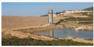
Boukhroufa Dam is under construction by Nurol Construction at the El Tarf province of Algeria. It is located on the Boukhroufa Stream, 9 km south of the Bouteldja city, to provide 125 hm<sup>3</sup> of irrigation water for agricultural lands in the region. The dam is a clay core earth fill dam and will be 87 m high from the foundation. Once completed, its reservoir will have 86,000,000 m<sup>3</sup> capacity.
