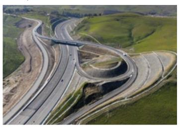
The 48 km long connection highway between Tizi Ouzou-Bouira in Algeria is operated by the Özgün-Nurol Partnership, and within the scope of the Project, 48 km of highway, a total of 2 x 1.670 meters of double tube tunnel, 21 viaducts, and other structures, infrastructure and drainage system manufacturing will be completed. The section of the Project between km: 0 + 000-10 + 000 has been opened to traffic, and the remaining parts are being constructed.
